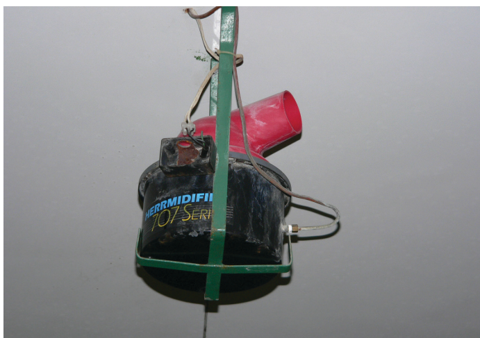
A storage room humidification unit
