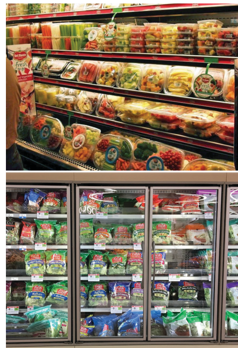
Figure 30. Open (above) and closed (below) refrigerated display cases. Credits: J. K. Brecht, UF/IFAS
