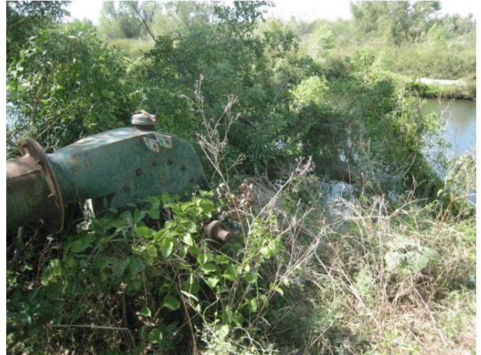
A pump used to extract water from the Rio Fuerte to irrigation canals
